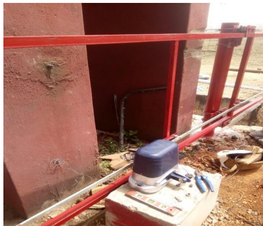
Figure 4: Rollers, gate, rack and motor in position.
